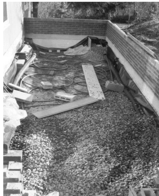
Figure 3 Water pre-heat coils in greenhouse
