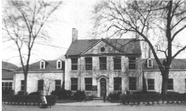
The Friendship House South Carolina Avenue façade as it appeared in 1951.
