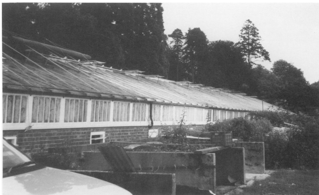
Figure 7. House VI, as it is today, seen from the south-west. The row of brick-walled bins containing compost etc., seen in the foreground, is on the site of the demolished House V
